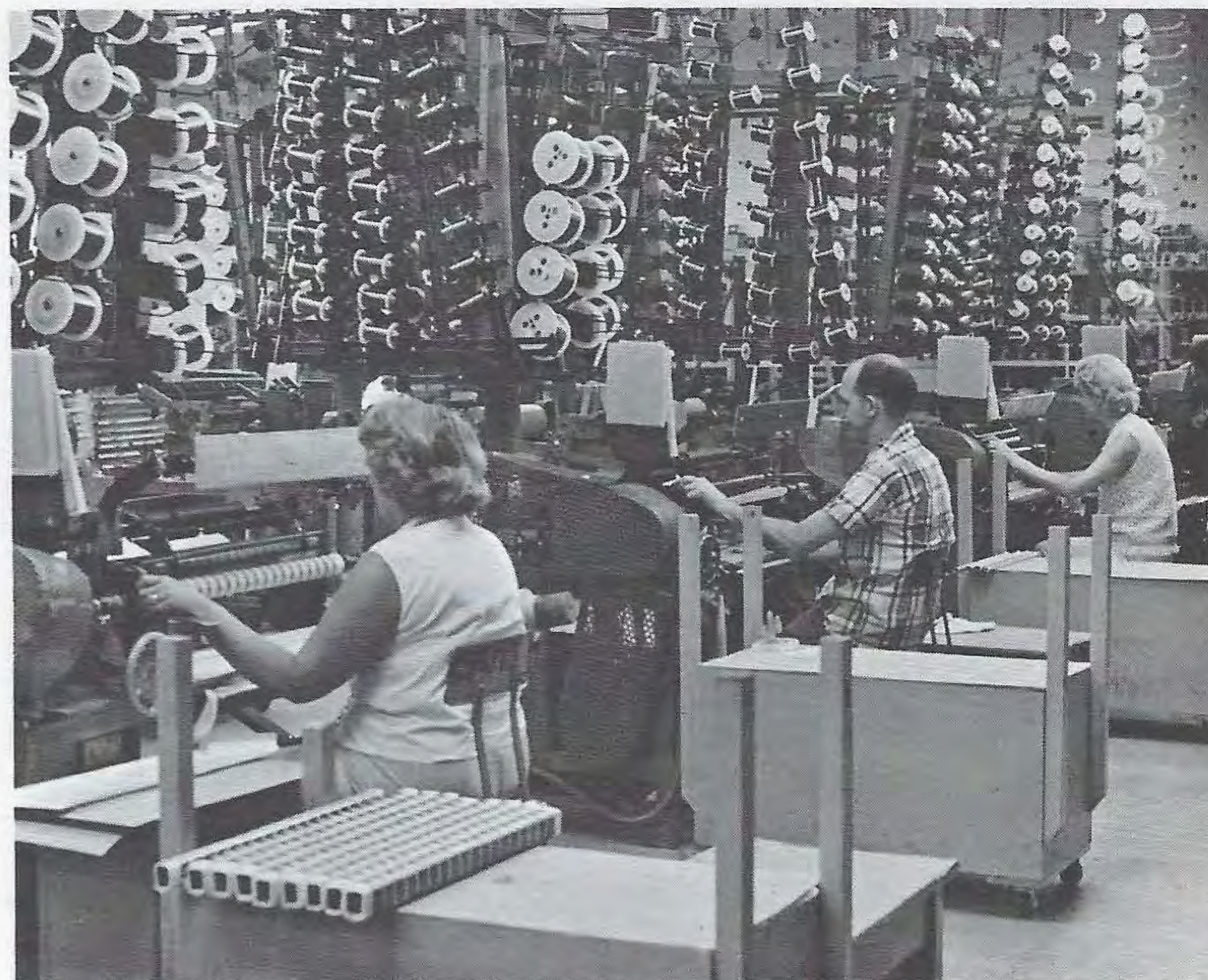
A view of some of the many multiple winding machines in Triad's Venice, California plant. The "Christmas tree" procedure dramatically cuts production time.
